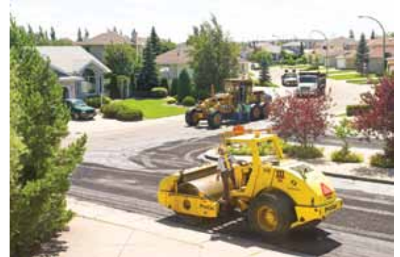
AP 00020-00-00-03 Neighborhood Road Work Paving (Saskatoon)
